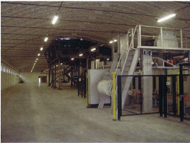
Bagging and palletising building.
